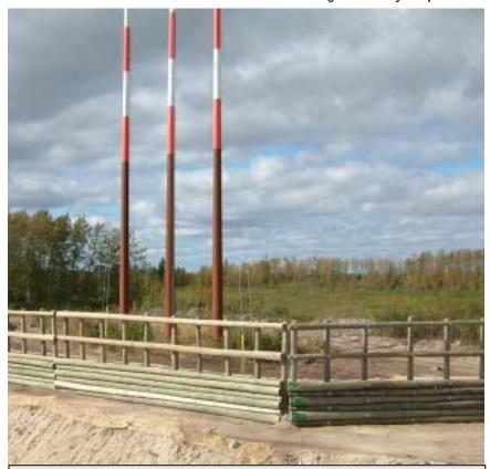
Berms have been built at major river crossings to protect the transmission line from damage at breakup d \a \d ` ^ ` " k [ c bV bd ` [ ; g ` ^j ` Al < ` ž \ ` bV @9 `j ` a ^< ` V c m " hc 0^ba \_l ` f b\J ` ž ` mj 0[ <B
